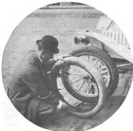
Fig. 1—First operation in adjusting Jenkins Emergency Wheel
